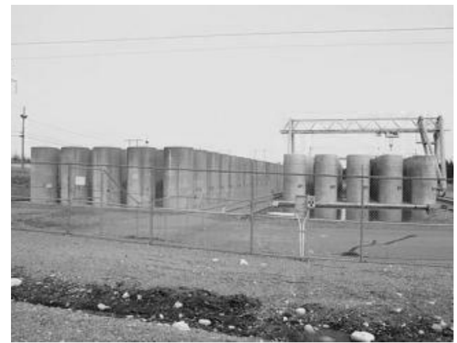
Aging concrete silos of deadly radioactive “high-level waste” produced by the Point Lepreau nuclear reactor on the Bay of Fundy. Photo from the CNSC.
